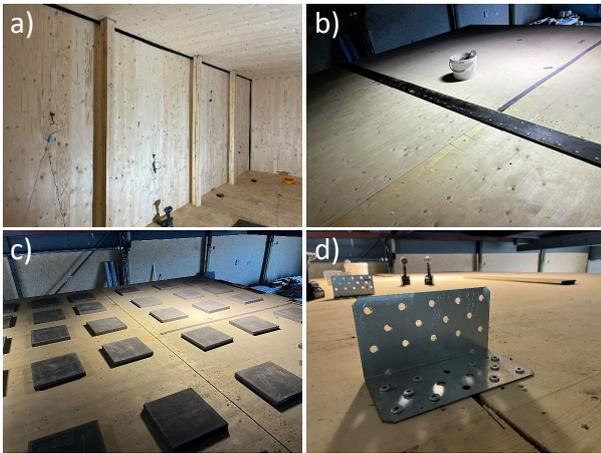
**Figure 4.** Photos of junction measures. a) Cut across roof and wall slabs (black line) and free-standing columns with sylomer RIs, b) chip board mounted across the roof slab cut, c) addition of mass to roof slab, and d) steel plates mounted across the roof slab.
